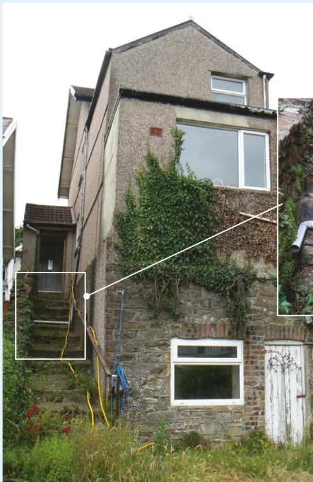
*In this home the accessway to the rear garden and garage is down a set of steep steps. These steps are in disrepair, slope dangerously and are slippery. The handrail is loose.*
