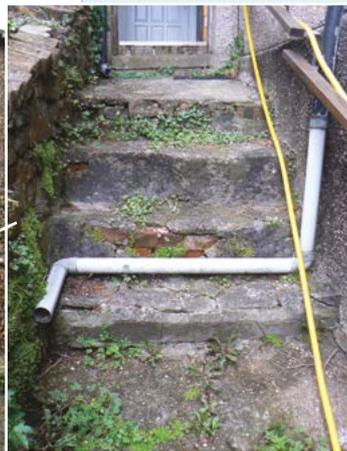
*To make matters worse, the rain-water drainage discharges directly onto the steps which means that they are always wet. Following a very cold night they would have ice on them. As this is a regularly used accessway this is deemed to be a Category 1 hazard to a vulnerable elderly person.*
